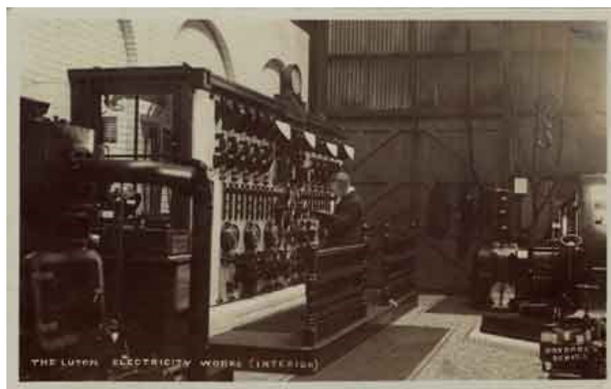
Luton Electricity Works, 1909 [Ref: Z1306/75/17/11]
